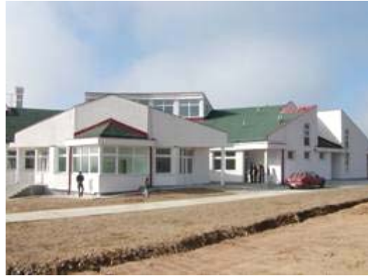
The school, the ambulance and the MZ (village council) now in the same place
