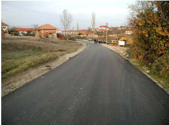
Rehabilitation of regional road Oslare – Nesalce
