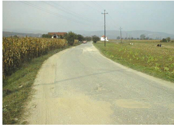
Internal road rehabilitation: Oslare – Levosoje
