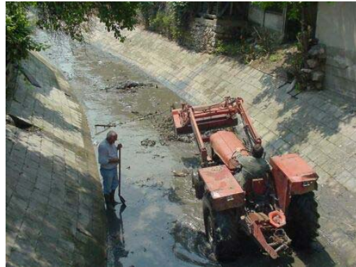
Public Works in Razanj: Cleaning of the local river
