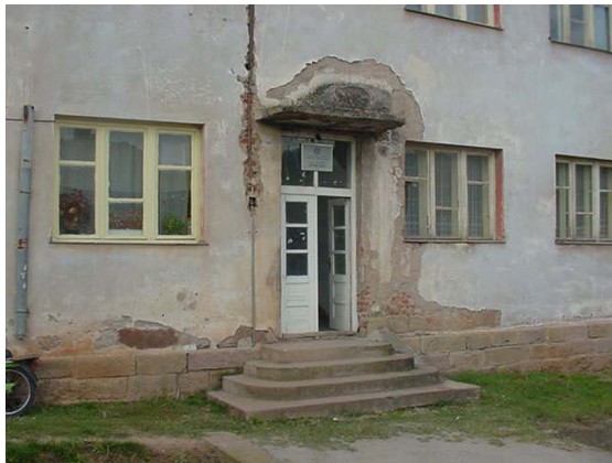
MZ Building before renovation
